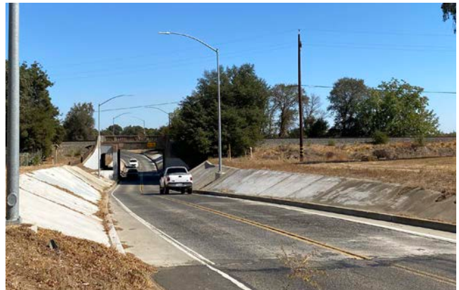
This Plan recommends the placement of 'Watch for Bicycles' signs on both approaches to the Union Pacific railroad underpass on Lower Sacramento Road, south of Woodson Road
