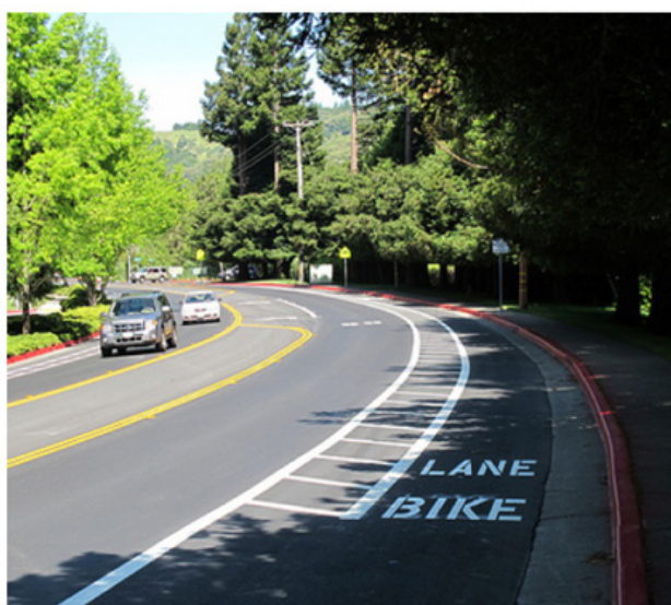
The use of pavement markings delineates space for bicyclists to ride in a comfortable facility.
