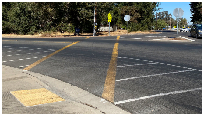
This Plan recommends the placement of advanced yield markings on both sides of the existing crosswalk at Thornton Road at Sacramento Boulevard and Oak Street, and upgrading the crosswalk to a marked crosswalk with vertical / painted bars
