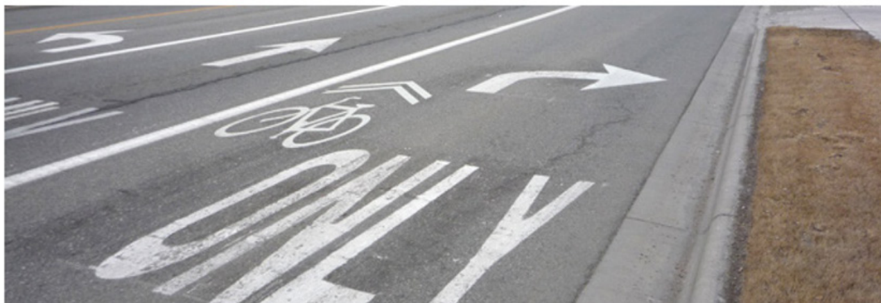
Shared lane markings and signs indicate that bicyclists should ride on the left side of this right turn only lane.
