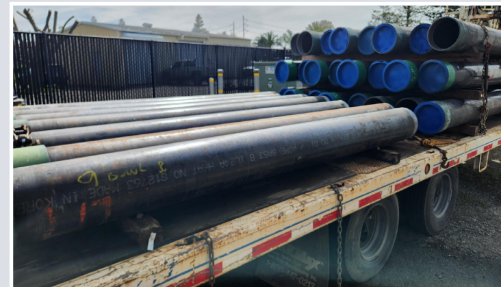
ARPA-Funded Well Improvements Project: After
