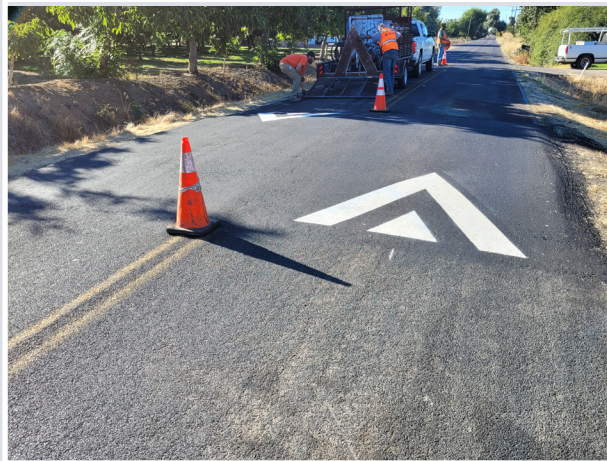
Speed Cushion Installation
