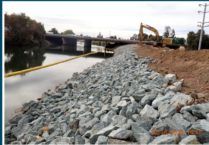
Calaveras River Erosion Control Project
