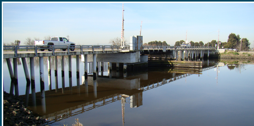
Movable Span Bridge Repairs
