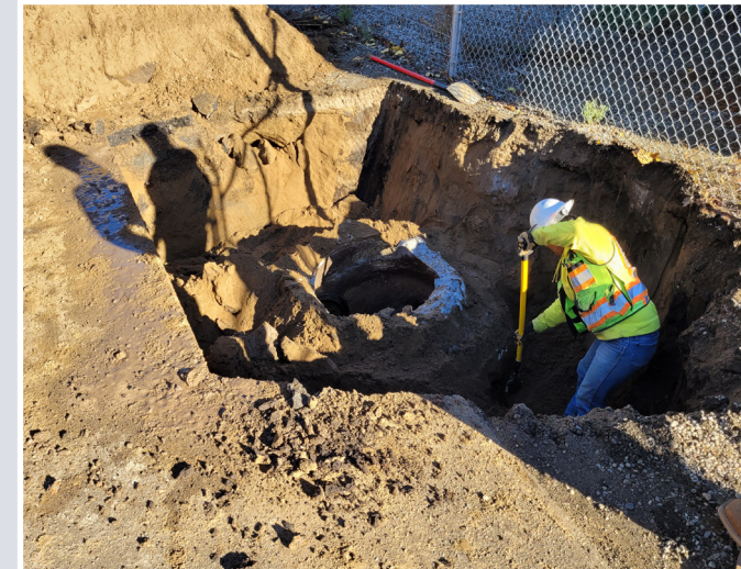
Pacific Gardens Sanitary District Sewer Project
