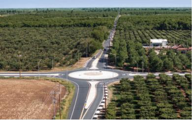
The project design team was tasked with designing a roundabout to accommodate extremely large agricultural equipment, including a 108-foot vehicle configuration.
