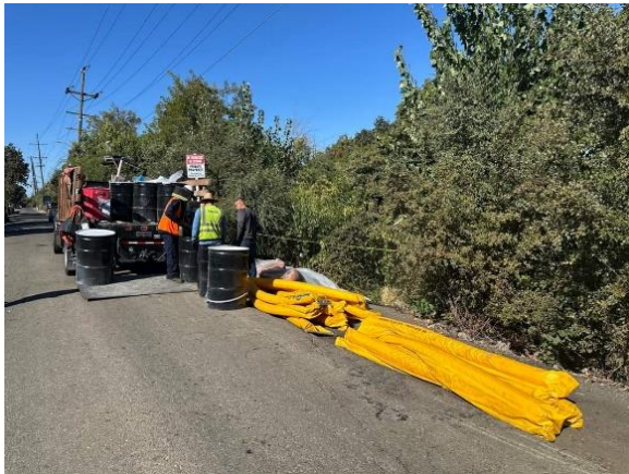
Crews continue clean-up and recovery operations on the Smith Canal.
