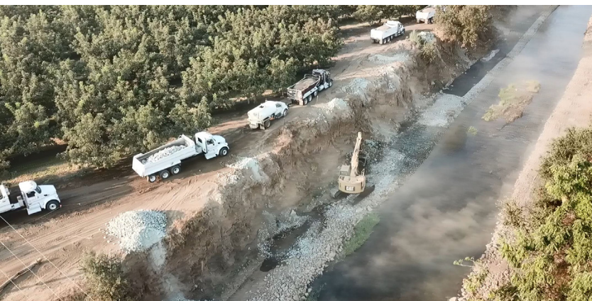
Upper Mormon Slough Erosion Repair Project
