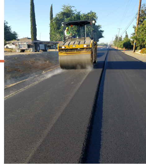
2021-22 roadway work from Public Works
