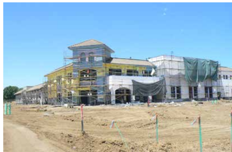
New Mountain House Town Hall Building
