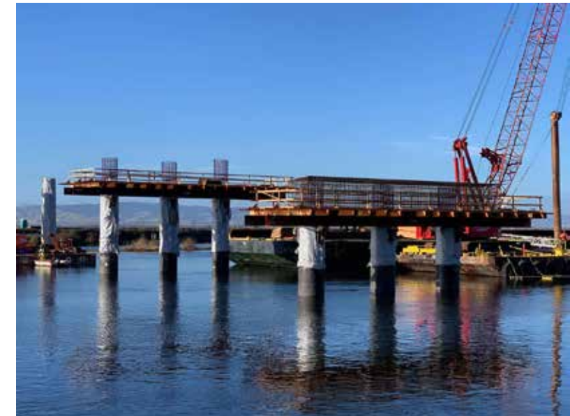
Woodward Island Bridge Construction (Photo by Bridgeway Civil Constructors, Inc.)
