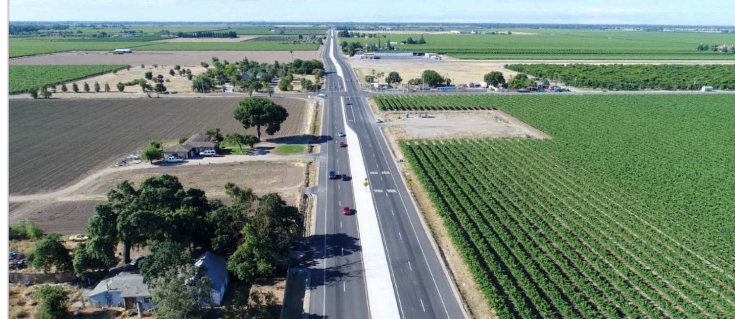
Lower Sacramento Road Widening Project
